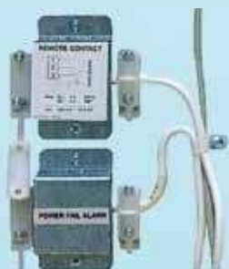
Remote temperature and power failure alarm
